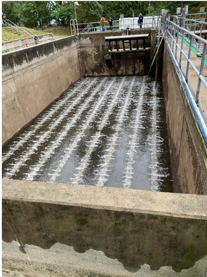
Inspecting the diffuser operation with clean water
