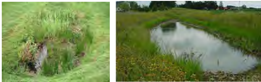
Stormwater infiltration ponds
