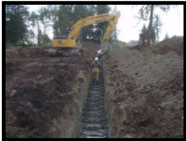
Beginning the installation of one of the Town's first geo-energy fields
