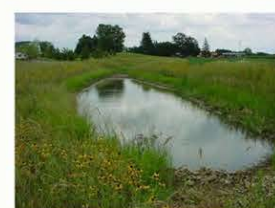
Narrow, curved stormwater infiltration ponds built into slope-fill progressively with stormwater volume.
