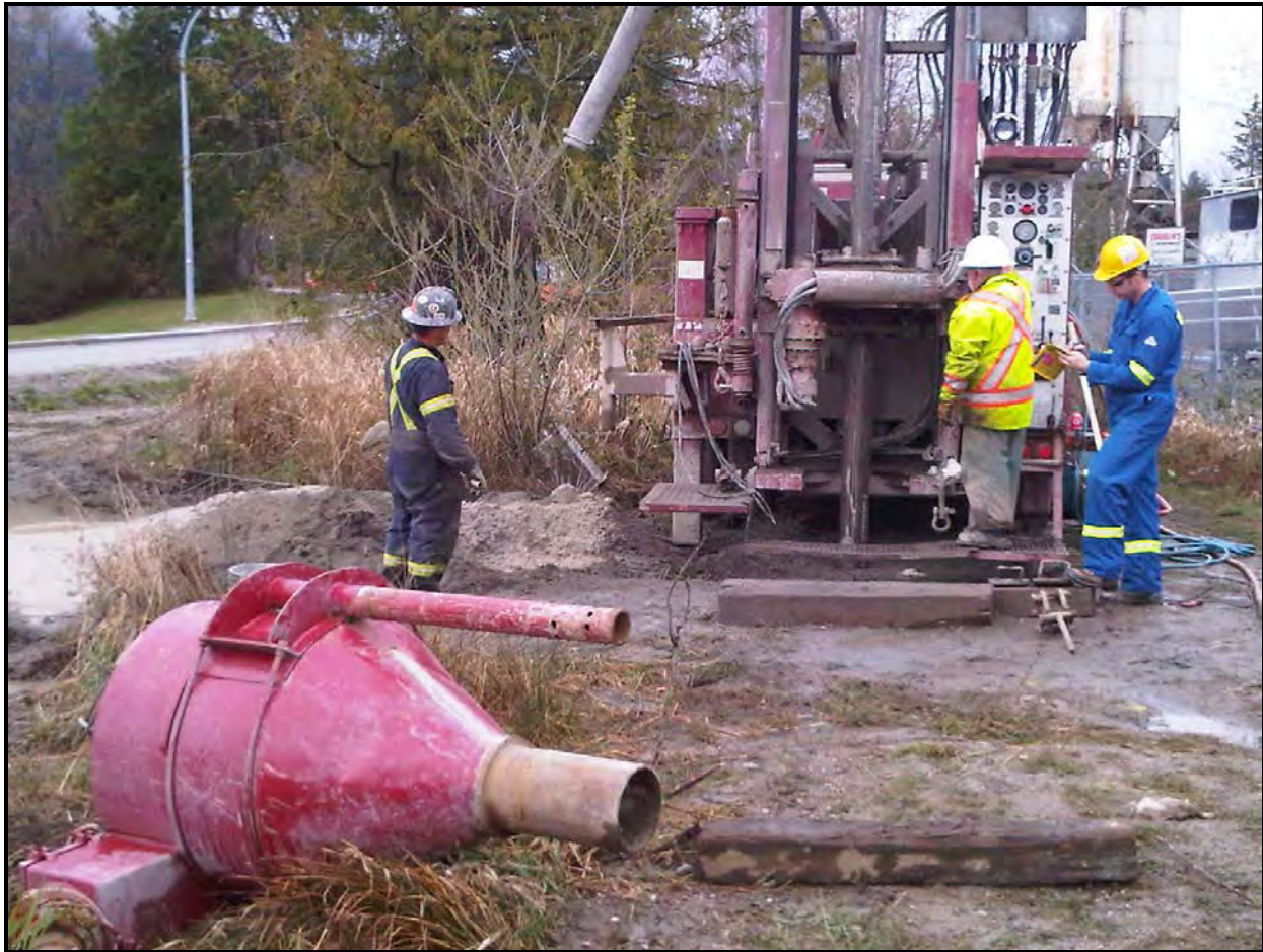
Figure 9: Photo of Drilling Operation at WL10-01
