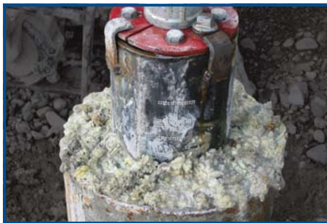
Figure 7. Bentonite cement grout seal between casings.
