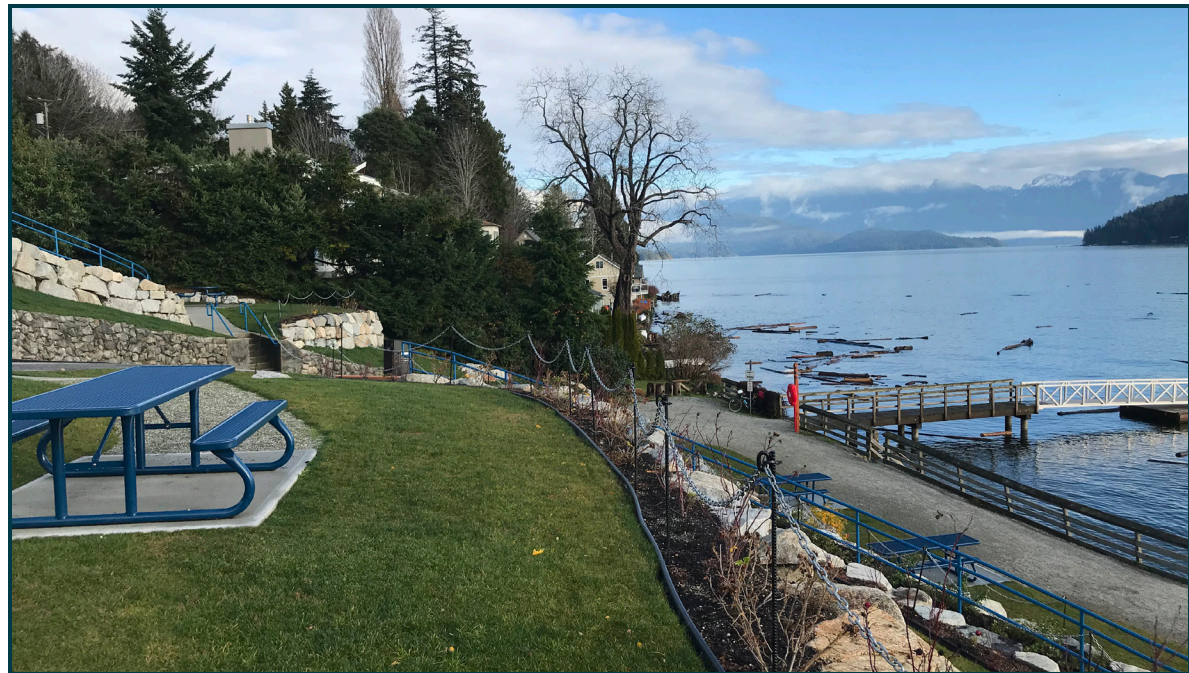
View of Armours Beach, following 2018 rehabilitation
