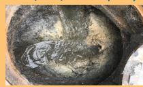
An annual flushing and monitoring program has revealed issues with preventable blockages, such as grease build up due to lack of grease interceptor control. In response, the Town has implemented a multi-pronged communications and inspection program aimed at both commercial and residential addresses.
