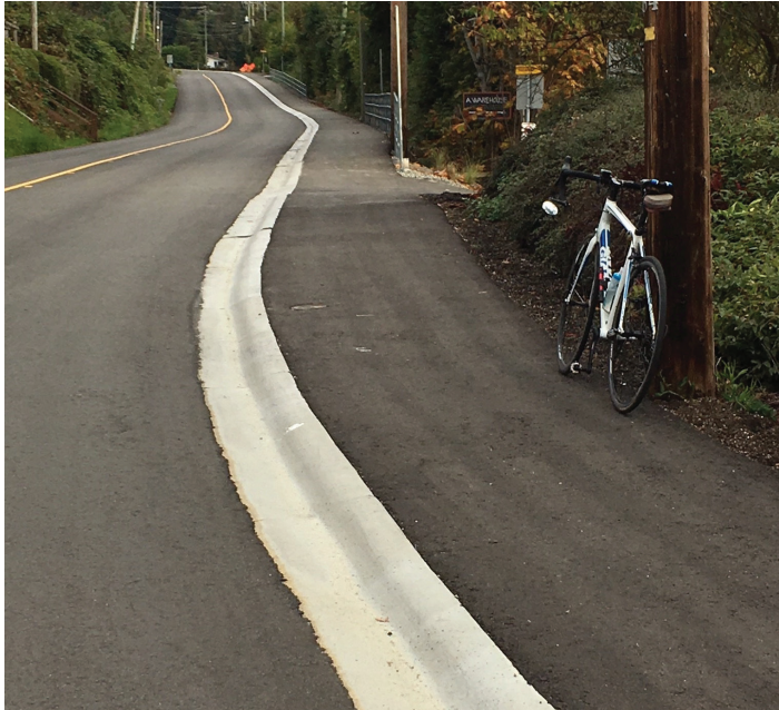
Gibsons Way Improvements Phase I - multi-use pathway on the west side of the downslope into Lower Gibsons.
