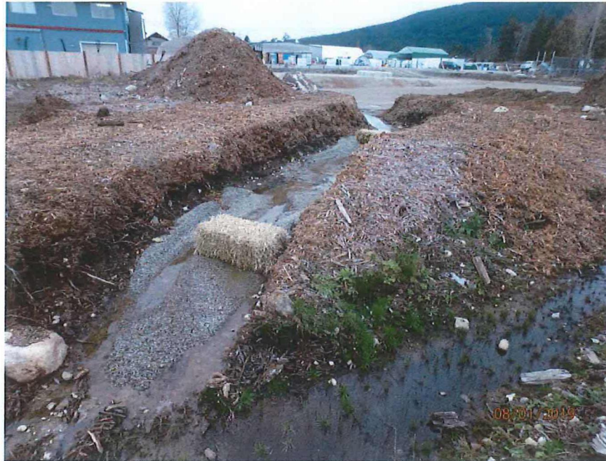
Picture 7 View to the northwest of the cleared lot at 1000 Venture Way. The recycling depot is in the background. Note some of the engineered drainage and erosion control measures.
