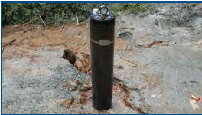
Figure 3. Erosion caused by flowing artesian well.
