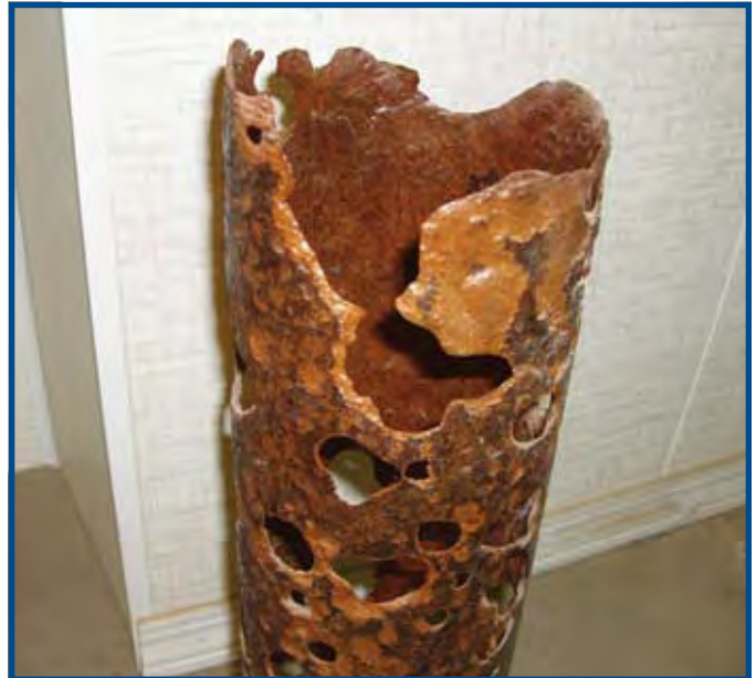
Figure 5. Corroded well casing.
