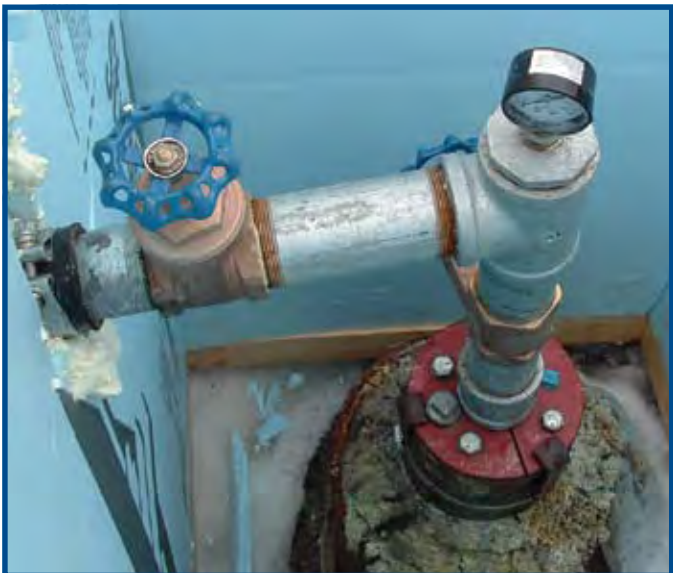
Figure 9. Completed high pressure flowing artesian well.
