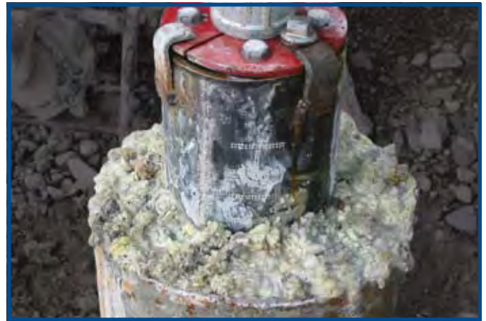
Figure 7. Bentonite cement grout seal between casings.
