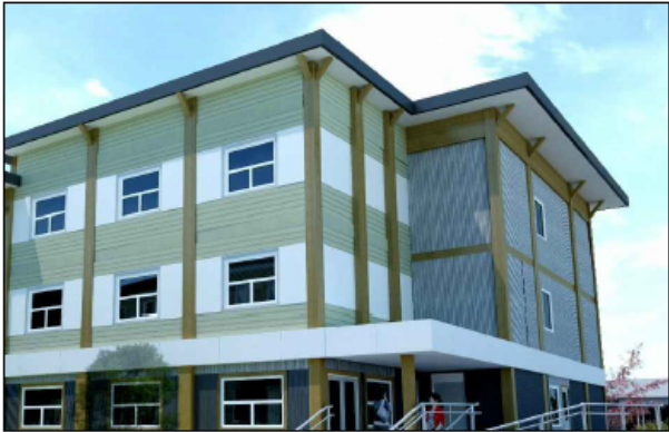
2. Fibre cement board panels and metal siding
