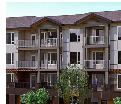
Sheltered exterior decks
