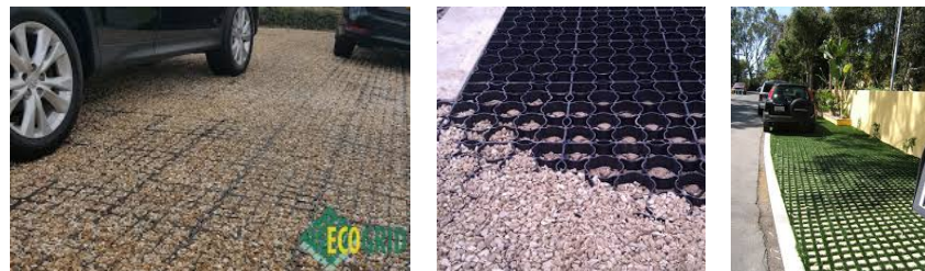
Permeable parking surface
