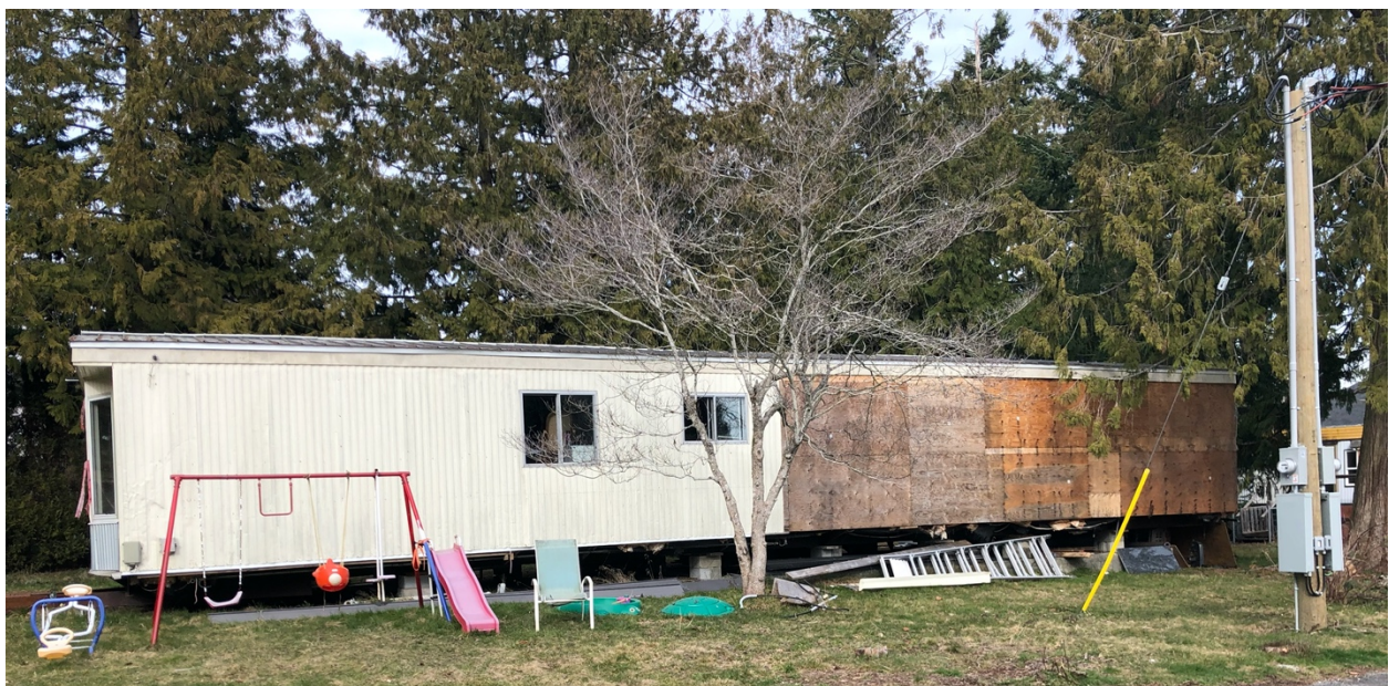
Figure 2: Derelict Mobile Home has now been removed from the sit. Photo taken February 21, 2020
