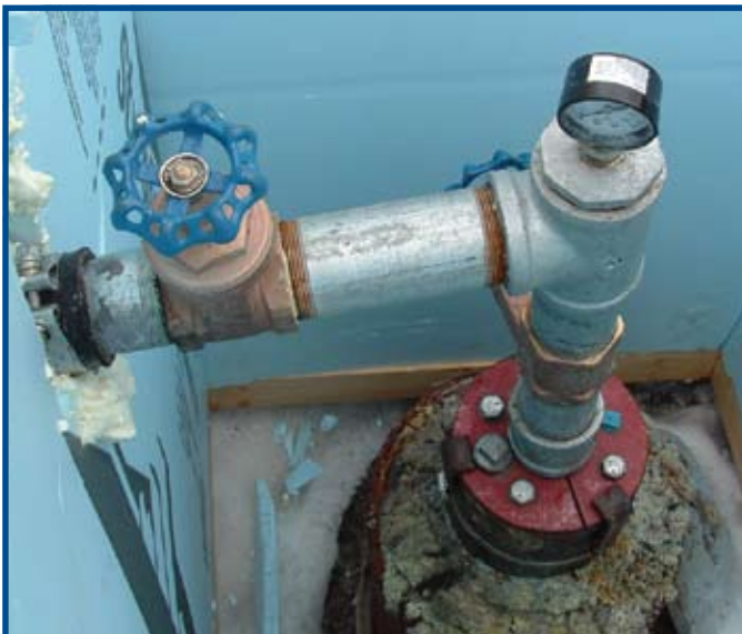
Figure 9. Completed high pressure flowing artesian well.
