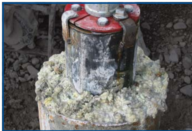
Figure 7. Bentonite cement grout seal between casings.
