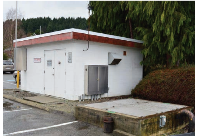
The Prowse Road Lift Station provides service for roughly 40% of Gibson's sanitary flows. Sewage from the eastern portion of the Town, which cannot drain by gravity directly to the wastewater treatment plant, drains to the Lift Station, and is then pumped via a force main to the wastewater plant for treatment.
