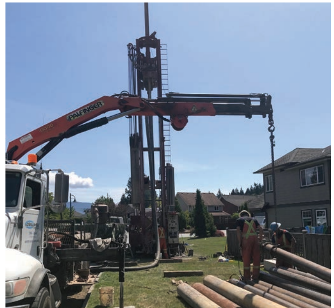
As a new supply well drilled in Dougall Park in early 2019 did not produce the amount of water required to expand the aquifer service into Zone 3, an additional supply well was drilled at the west end of Oceanmount Blvd. This well has proven to be an excellent producer.
