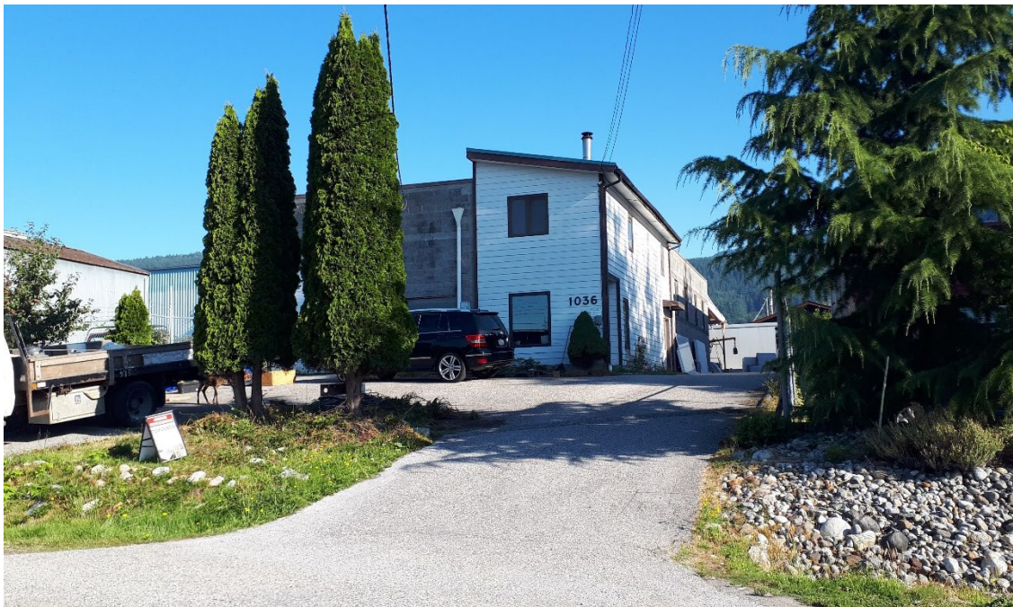
Figure 2 - Existing building (August 2020)
