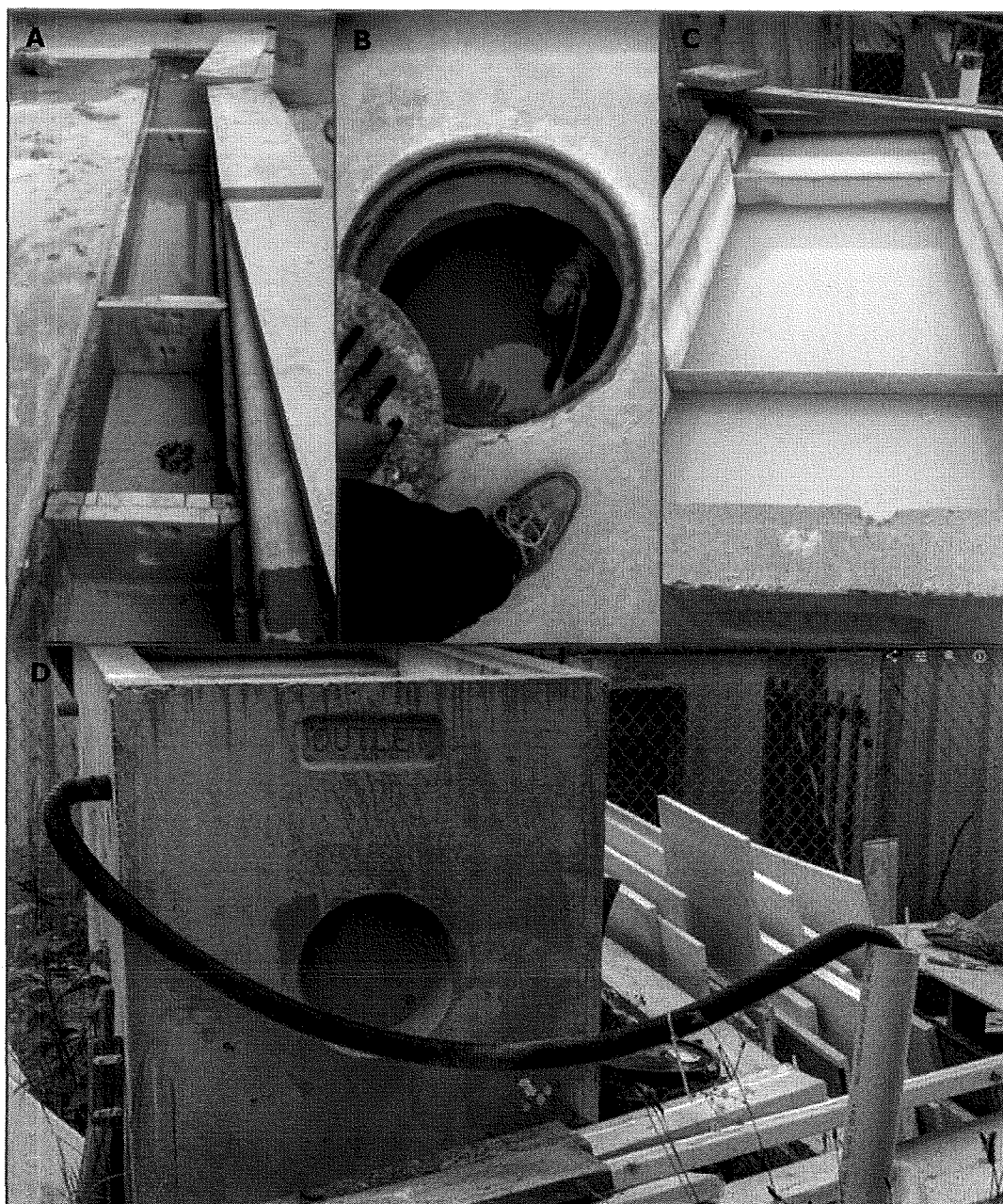
Figure 5. Wastewater management system of the current facility. Wastewater generated during manufacturing and polishing activities drains from working areas into perimetral concrete trenches and sedimentation traps under the main floor ( A ; trench covers removed for illustration purposes) draining into a centralized collecting and sedimentation well ( B ). From the collection and sedimentation well, wastewater is pumped into a secondary three-stage sedimentation trap ( C and D ). Wastewater from the sedimentation trap is release into the Town of Gibsons sanitary sewer system ( D ).
