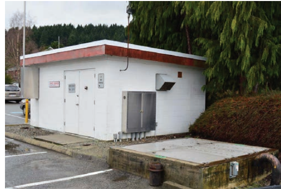
The Prowse Road Lift Station provides service for roughly 40% of Gibson's sanitary flows. Sewage from the eastern portion of the Town, which cannot drain by gravity directly to the wastewater treatment plant, drains to the Lift Station, and is then pumped via a force main to the wastewater plant for treatment.
