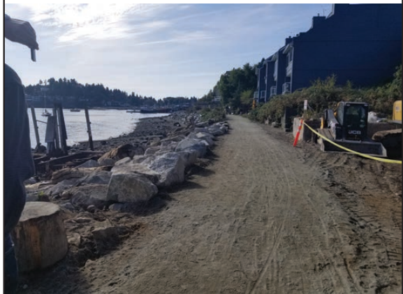
Improvements in front of the old Coles Marina site built up the area over the trunk sewer to provide a continuous level area for maintenance vehicles and pedestrians.
