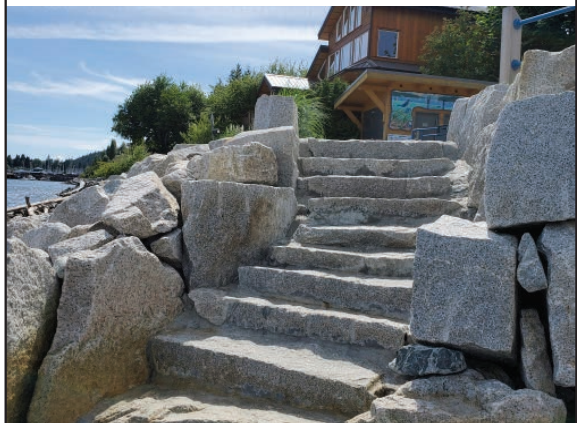
The improvements in front of Armours Beach included replacing a failing block wall with sloped rock protection and rebuilding the stairs down to the beach.
