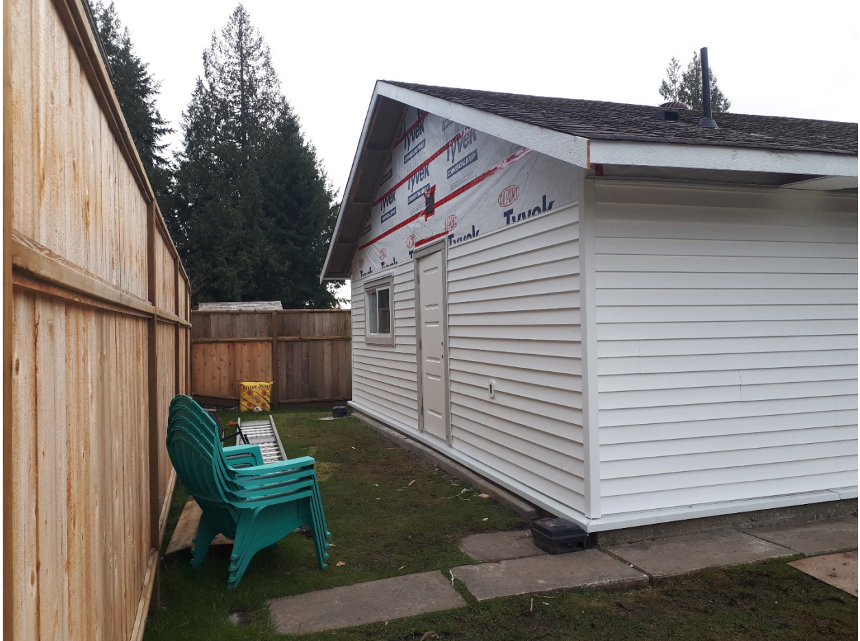
East side view with secondary exit door and new siding in progress. Fences on east and south property lines screen view of suite from neighbours. Clutter is related to building in progress under existing building permit.
