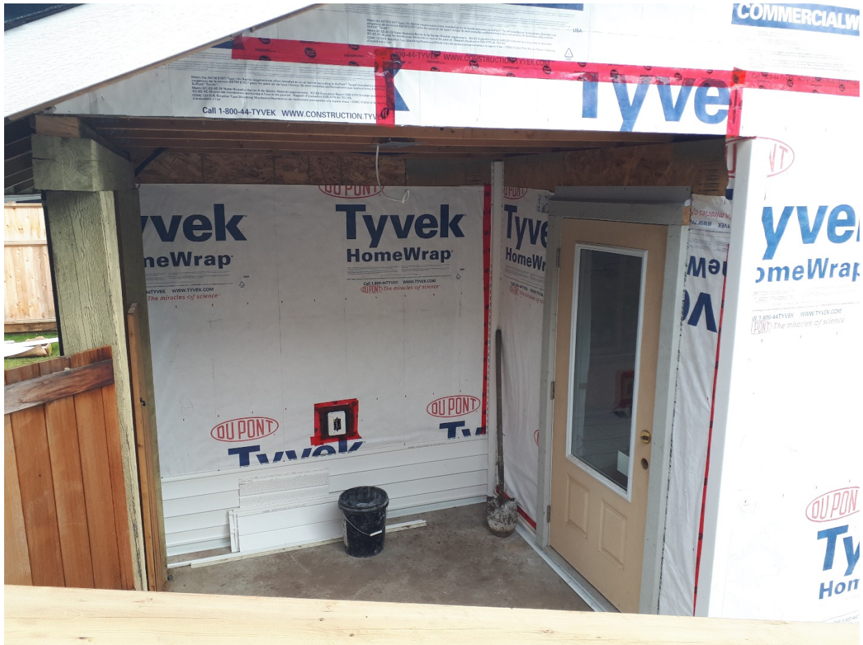
Main entry alcove with new front door and new siding in progress (northwest corner of suite). Photo taken from temporary accessibility ramp to main dwelling, to be removed.
