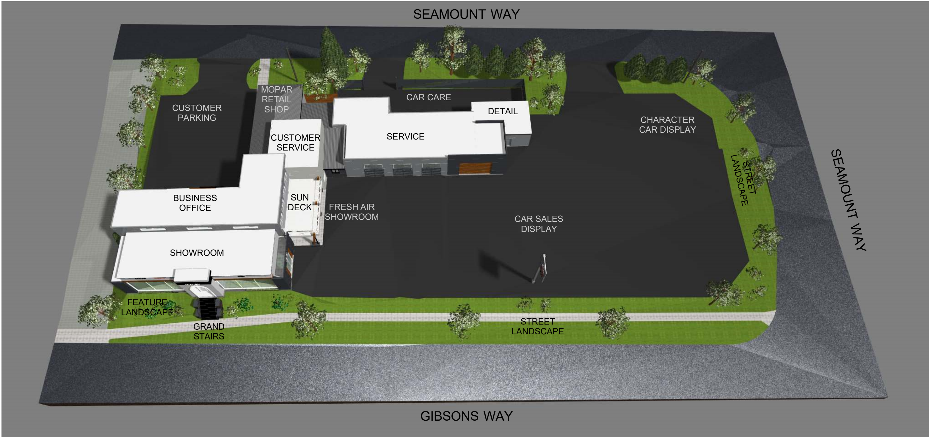
SOUTH AERIAL IMAGE
