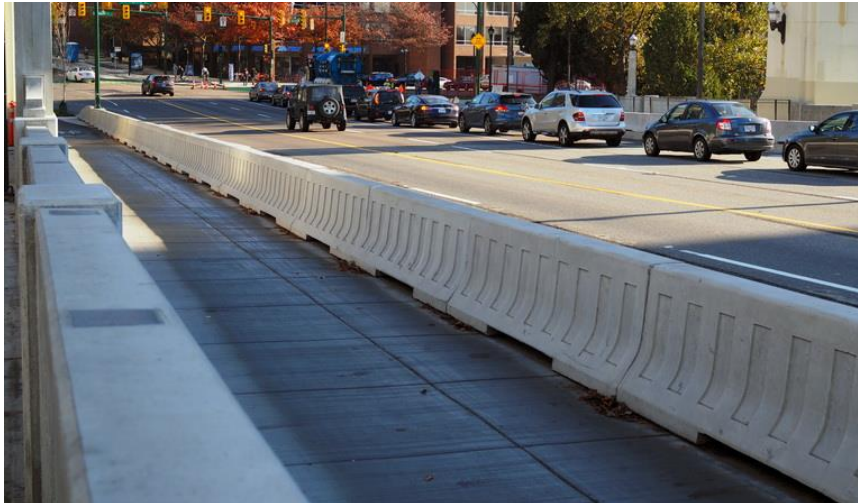
Figure 3: Patterned Precast Concrete Barrier – Burrard Street Bridge (Vancouver, BC)
