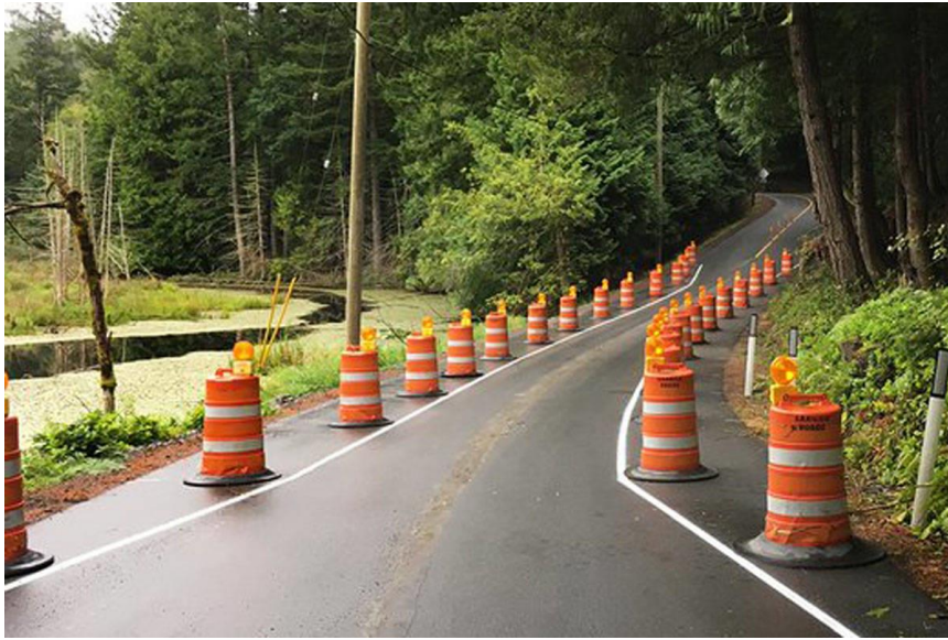
Figure 2a: Temporary Single-lane Road Segment (Prospect Lake Road – Saanich, BC)
