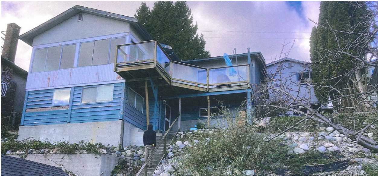
Figure 4 - existing deck to be replaced.
