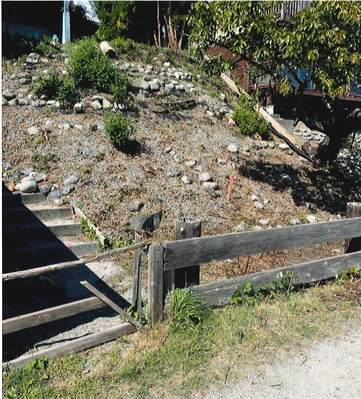
Figure 1: Current state of rear yard slope, looking west from waterfront path. Wood stakes with orange flagging delineate property boundary.
