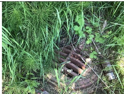
Photo 6. Stormwater drainage ditch along west side of Shar road at northeast lot corner. Water table approx. 1m below road surface during observation.
