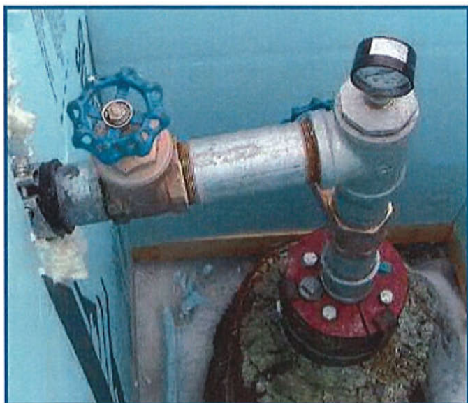
Figure 9. Completed high pressure flowing artesian well.
