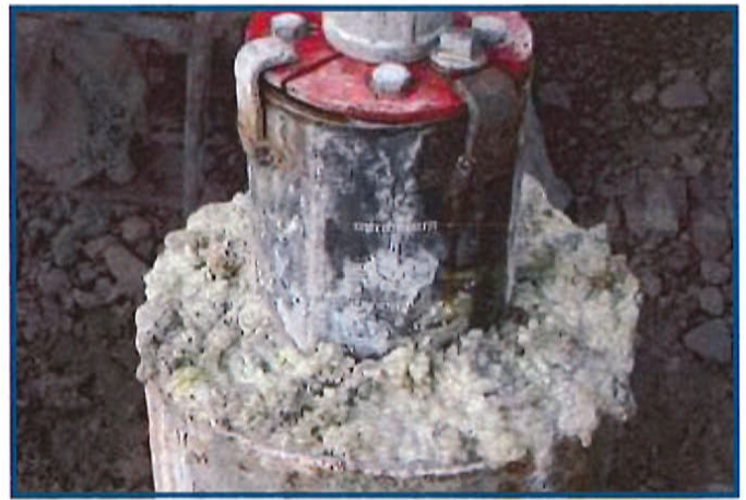
Figure 7. Bentonite cement grout seal between casings.
