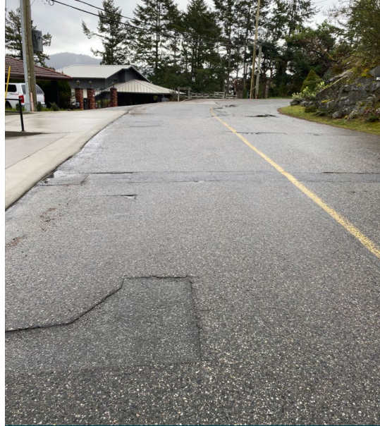
Skyline Drive Water Main ($2.185M)
