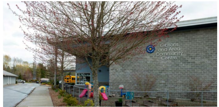
700 Park Road (Gibsons and area Community Center)
