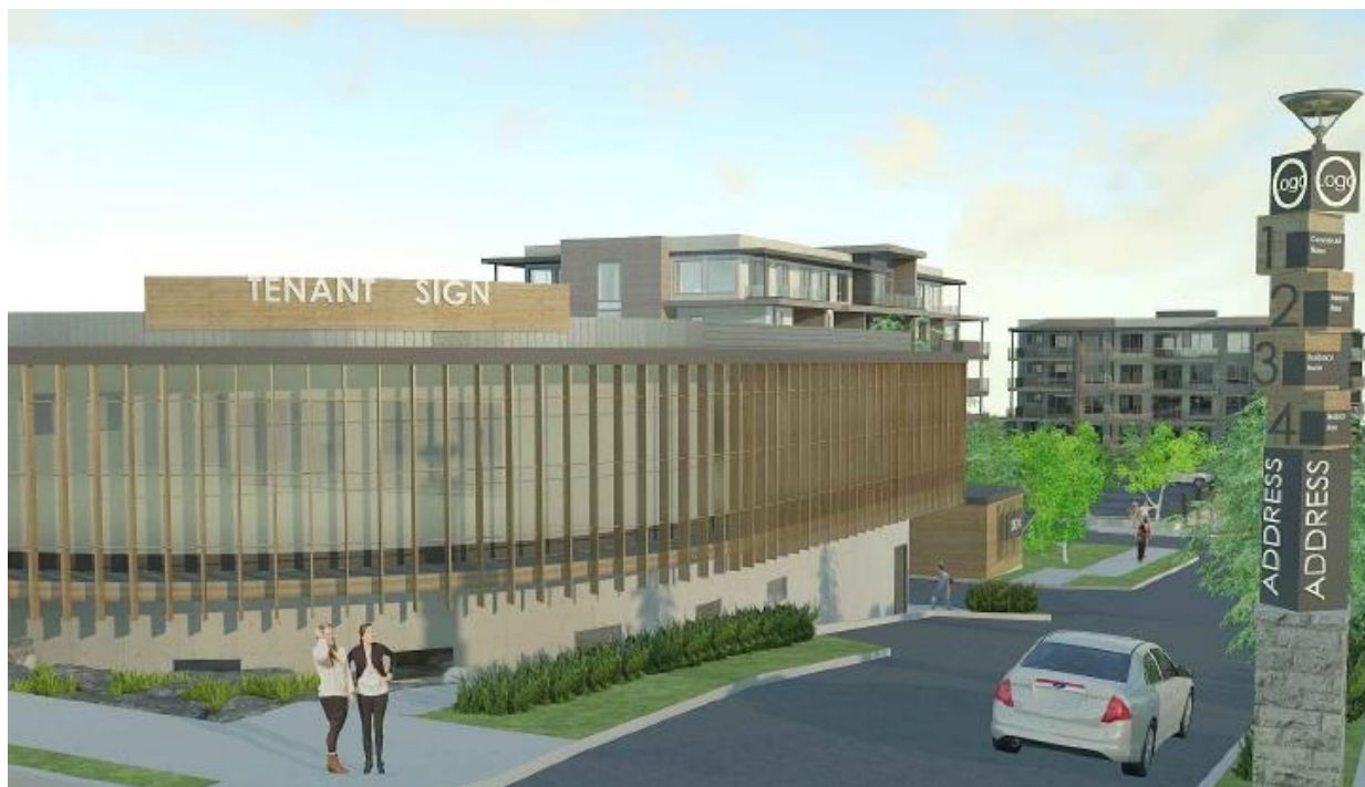
Figure 3: View of development from entrance on Gibsons Way, showing building A
