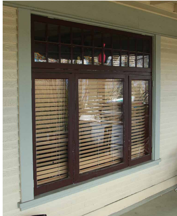
Tripartite casement window with awning style multipane transom above at porch level, 2024. [Donald Luxton & Associates]
