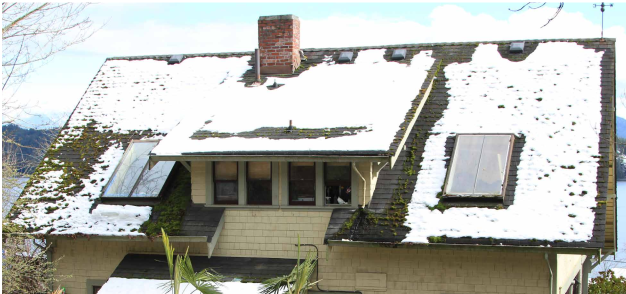
Rear wall dormer with shed roof. Side skylights are not original to the building. [Donald Luxton & Associates]
