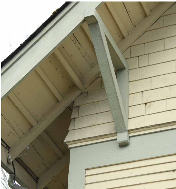
Condition of wood trim elements: triangular knee bracket, exposed rafter tails, pointed bargeboards, 2024. [Donald Luxton & Associates]
