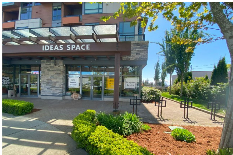
Image 2. Bike parking and shelter at the front entrance of buildings.
